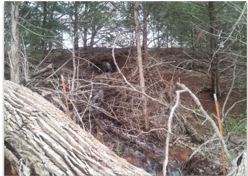
Hole & seepage of a dam in Oklahoma City
