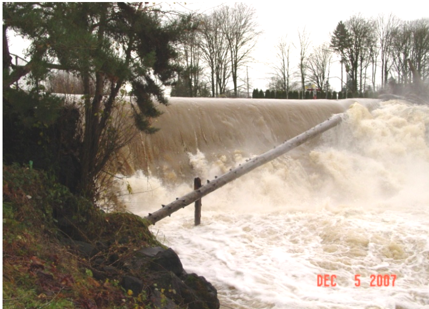
Overtopping of Tumwater Falls Dam, Washington
